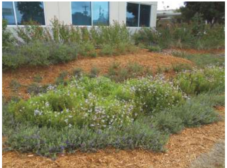
The River Authority Environmental Center bioretention area includes a rain garden to help capture stormwater runoff.
